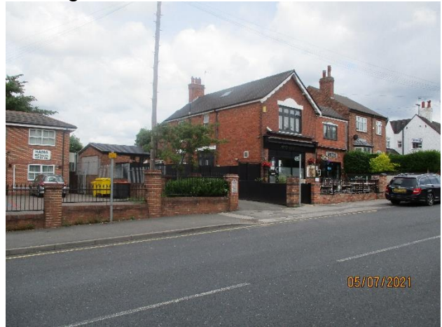
View of garage to be converted from Nottingham Road.
